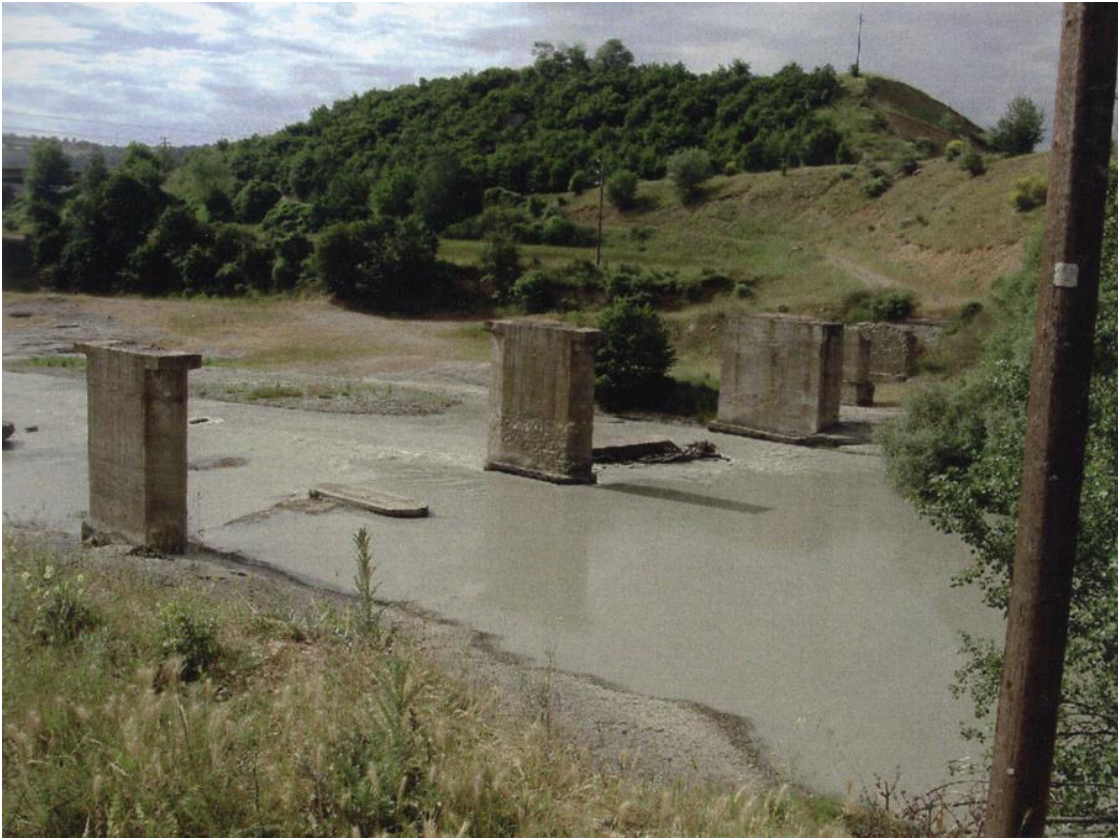
Figure 2 – The remnants of the Aliakmon river bridge (aka “Pasha’s bridge”).
